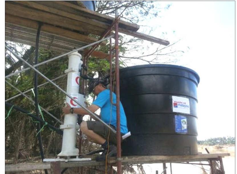
*Setting up a SkyHydrant water filter properly will ensure that it lasts its expected lifespan of 10 years or more. Here, dirty water will be fed from above and gravity will push it through the filter into the adjacent container. Up to 1,000 litres per hour of filtered water can be delivered.*
